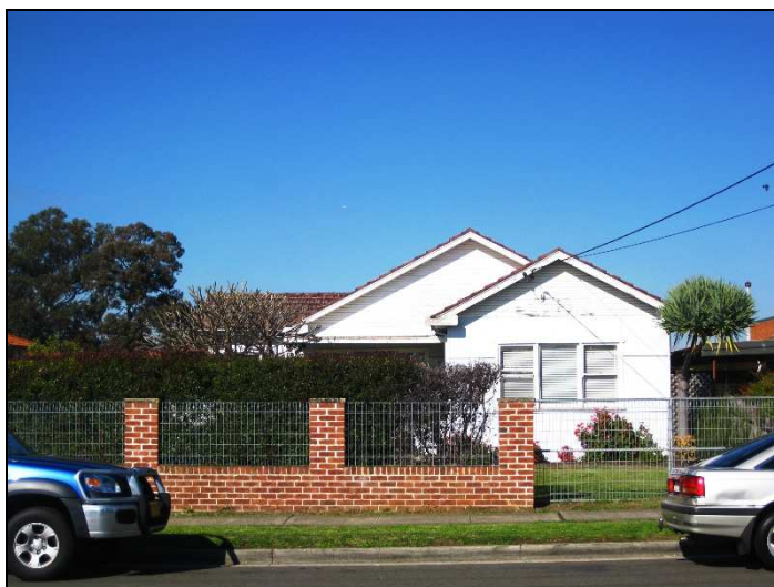
Photograph 1: Subject Site (No.131 Polding St) viewed from across the road looking south
